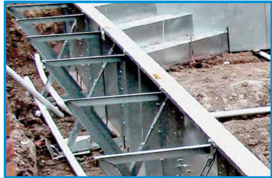
THE TRIDENT STEEL WALL PANEL AND BRACE SYSTEM
